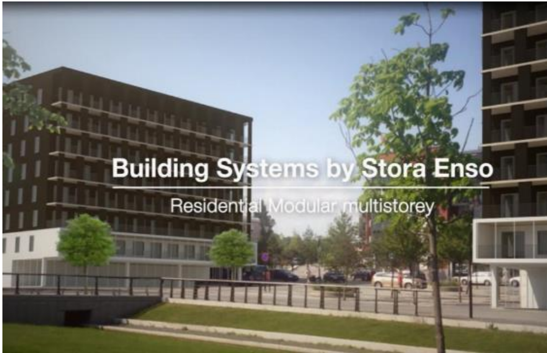
Residential multi storey panel construction
