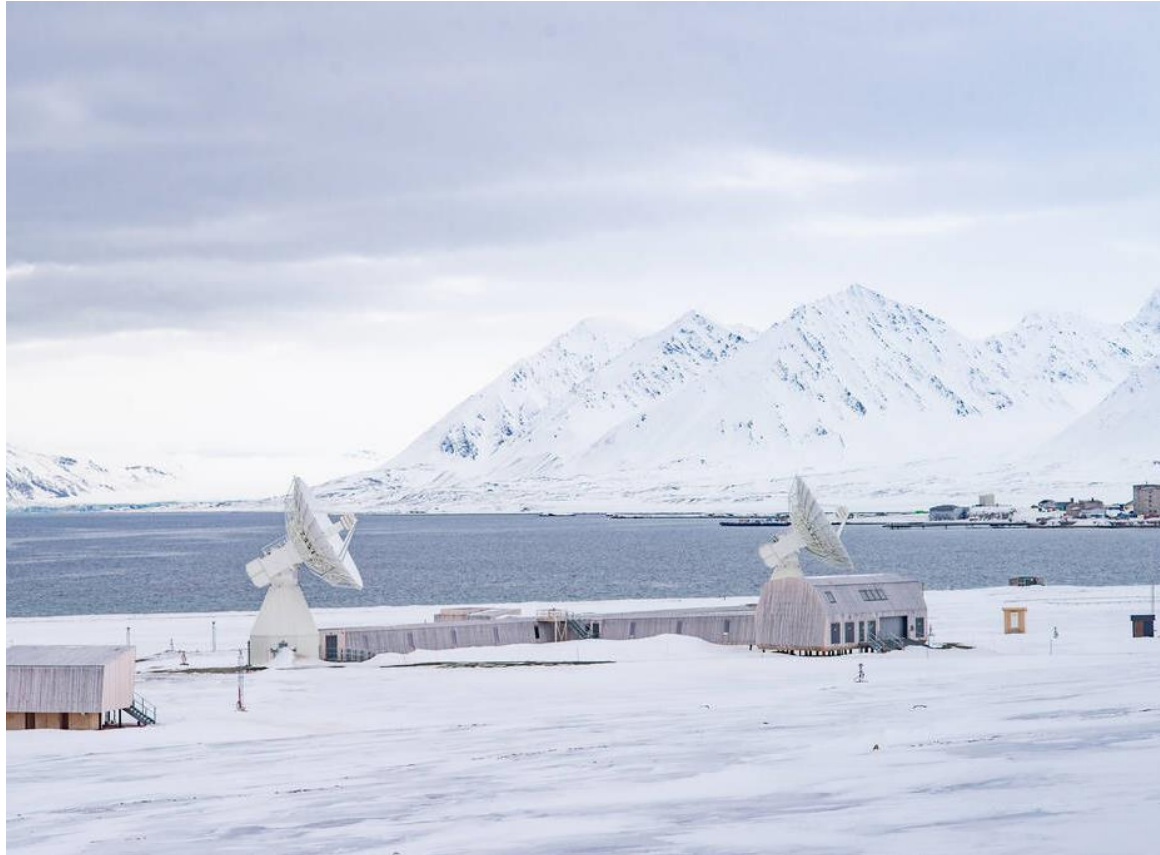
Earth Observatory, Geological Research Base on Svalbard Norway Cross Laminated Timber floors and roofs by Stora Enso
